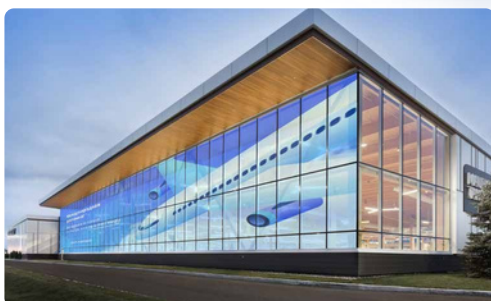
BUILDING CURTAIN WALL
